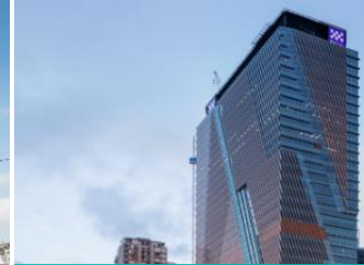
Jul 2020: Completed Victoria Police Centre in Melbourne
