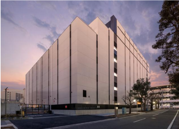
Tokyo Data Centre 3
