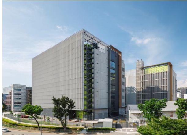
Keppel DC Singapore 7 & 8
