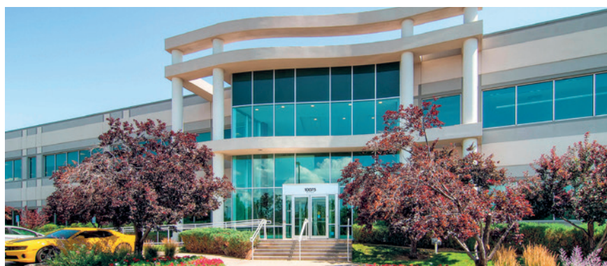
Westmoor Center, LEED Gold Status
